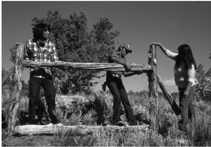
Rudy Hammond supervises students learning how to build fence.
